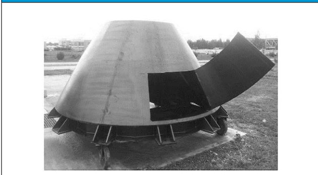
Fig. 12. Base concluded. Source: Authors
